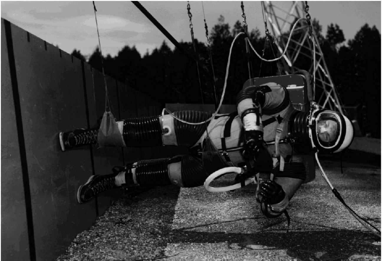
*Researchers at Langley Research Center studied astronauts' ability to walk, jump and run using this ingenious lunar-gravity simulator. The astronauts wore pressure suits that were supported by a system of slings, cables and a trolley that was controlled by the subjects as they performed maneuvers. The facility also studied astronaut fatigue limit and energy expenditure in the one-sixth Earth-gravity conditions.*
