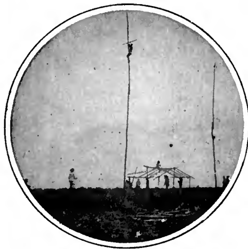
ERECTING WJS'S MASTS
