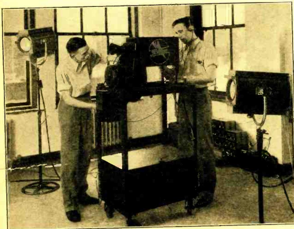
Students setting up the scanning apparatus of a television transmitter. The model shown televises the features of a direct-lighted human subject.
