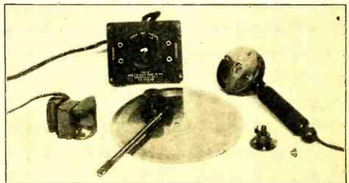
A complete kit of parts for use with any radio-phonograph combination; this includes a heavy recording head (leather V-way at left of needle-holder); hand microphone; ungrooved Emerson-Wadsworth double-faced record blank; feed-rod and center-post clamp; end-rest; and, in the background, the 4-way circuit-changing switch-box, provided with tip-jacks for recorder and microphone leads.
