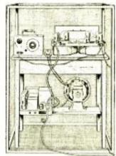
aligning cage, recommended by them. Though powerful station broadcasting on 1,260 kc. might cause enough interference to prevent correct align-ment of the set at the 1.264-kc, point, an aligning cage can be used effectively in a service shop, as at the factory, to reduce this interference, and it will permit accurate alignment of the instrument in the shortest possible time.
