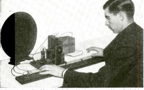
A photograph of one of the Editors testing the Trautonium. Tones are generated by moving the index finger of either hand along the manual.
