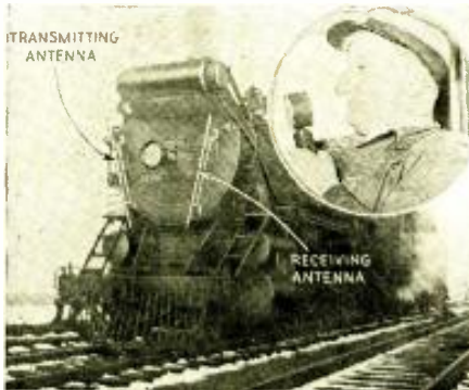
THE RADIO FREIGHT TRAIN To ease the difficult job of the engineer and brakeman on those mile-long trains.
