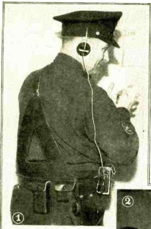
The individual police receiver shown above heralds in a new era in police radio. The instruments shown at the right demonstrate how ultra-short radio waves can be transmitted through water. If experiments verify the expected results, it will be possible to increase the range of transmission on these waves which are limited now to a maximum of about 100 miles. The towers at the lower left support the parabolic reflectors of the 17.8 centimeter transmitter and receiver. The portable transceiver in the lower right is used for fire fighting.
