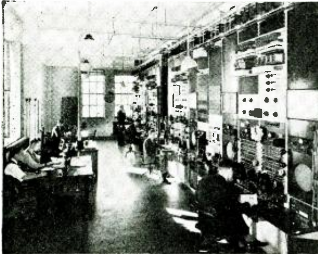
General Control Room, N. Y., supervises the nets. (Bell Tel. Co.)
