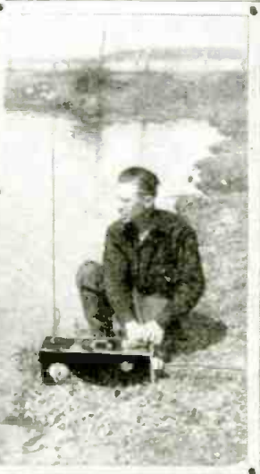
← RADIO-CONTROLLED MODEL BOAT. Felix La-Vallee, a Minnesota farmer, built this boat which he operates on a nearby lake. The controlling board of the ship is shown at left. The boat can be started, stopped, or turned by tapping the key. (World Wide Photos)
