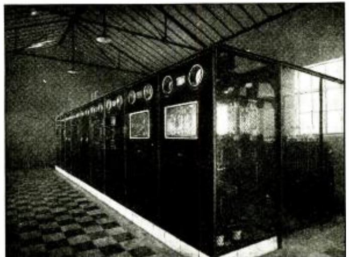
The radio telephone station at Buenos Aires, Argentine, used for commercial telephone communication purposes.
