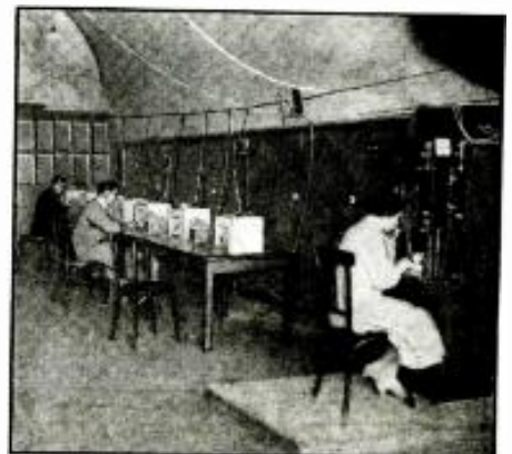
A section of the French reception center with switch-board to the Postmaster's office.
