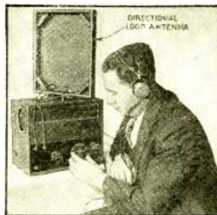
Fig. A. The loop points toward the station.
