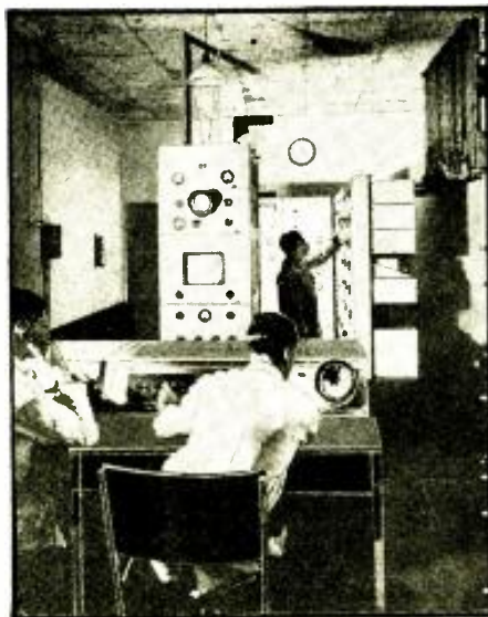
Control room and amplifier racks for the Baird installation at Alexandra Palace. Note the monitor cathode-ray image tube on the control desk (right) and the acoustically treated walls and ceiling. The Baird installation is alternated with the Marconi-E. M. I. system. Each station is usually on the air one day while the other is silent.
