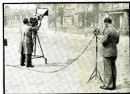
The mike may be clipped into the back of the 4-unit loudspeaker or may be used at a distance. All power is obtained from a 12-V. storage battery. It's hard to duck this word barrage!
