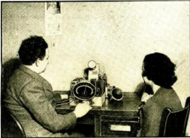
Fig. 8. Mr. Sobel with his version of the RADIO-CRAFT vision receiver. The set is housed in a "table" cabinet laid on its back.
