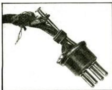
Here's an interesting sample (first shown in *Sylvania News*) of home-made service work. "We took this speaker plug out of a set that came in for service. The only trouble was that the wire wasn't making good contact with the nail!", says Broun D. Rinehart, Rinehart Refrigerator and Radio Sales.
