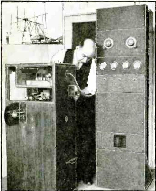
Fig. E. Checking-up the 6-V exciter lamp. Insert—experimental television news service antenna.
