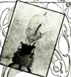
Edison's Incandescent Lamp with Plate Element. Responsible for Discovery of Edison Effect. TAE
