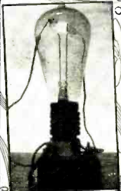
Edison's Incandescent Lamp with Plate Element. Responsible for Discovery of Edison Effect. TAE
