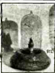
Fleming Valves or 2-Element Tubes, 1903-7
