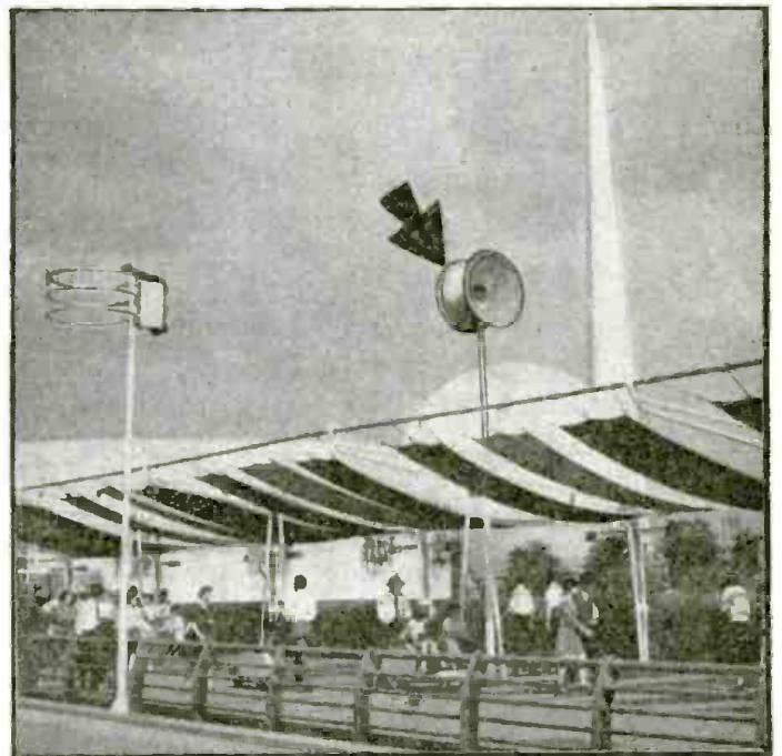
▲ One of the many loudspeaker outlets at the New York World's Fair; the perisphere and trylon theme in the background adds an artistic touch to this view. A single Cinaudagraph cone-type loudspeaker is mounted in a double baffle so that both front and rear sound waves of the speaker are utilized. (The 3 circles shown on pole at the left are decorative lights.)
