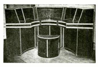
In some cases the lower compartments may not be used at all, in which case it is not necessary to have any holes through the table tops F. However, when leads are run from under the hood down to the lower compartment, it is of course necessary to cut through table top F and the corresponding lower half; this is readily accomplished with a wood bit, or for larger openings with an expansion bit or a keyhole saw.
