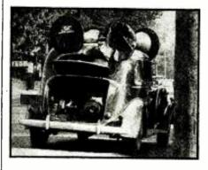
ORDINARY automobile spare-tire covers were put to a novel use by a California radio dealer. He found them to be just the right size and shape to fit over the end of the loudspeakers used in his public address system, protecting them from the rain, snow, etc., when not in use.
