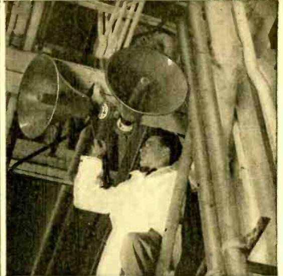
Above—Two of the Atlas Sound DR-42 Dynamic Reflex Projectors installed in the Pratt & Whitney Aircraft engine assembly building. There are 3 speakers in the cluster, one being hidden by the column.
