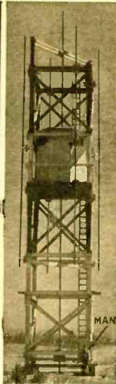
*This apparatus gives a visual indication of the direction of regular communication signals sent from a plane, and permits the flying field and the pilot to ascertain the position of the plane at any given moment.*
