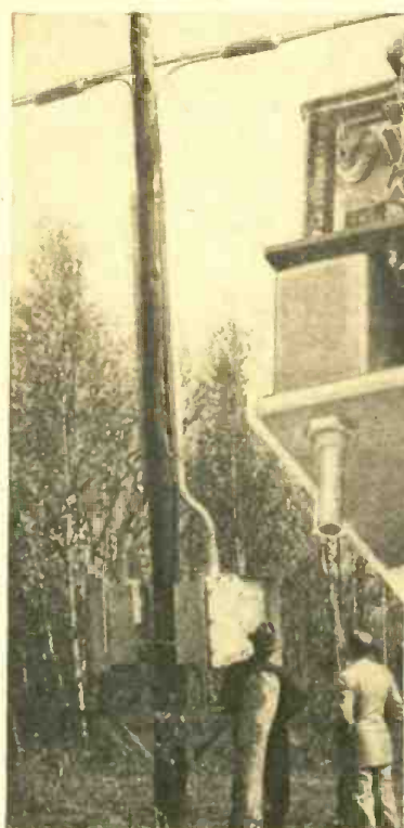
The picture at the left shows repeater station mounted in a weather-proof cabinet on poles—one method of mounting repeaters. Above: Close-up of one of the high frequency amplifiers used for L-1 carrier system, operated over the coaxial line here described.
