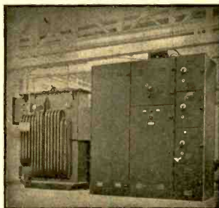
Sealed ignitron rectifier of factory-assembled load-center unit-substation type, installed in a large war plant. 300-kw, 250-v size.
