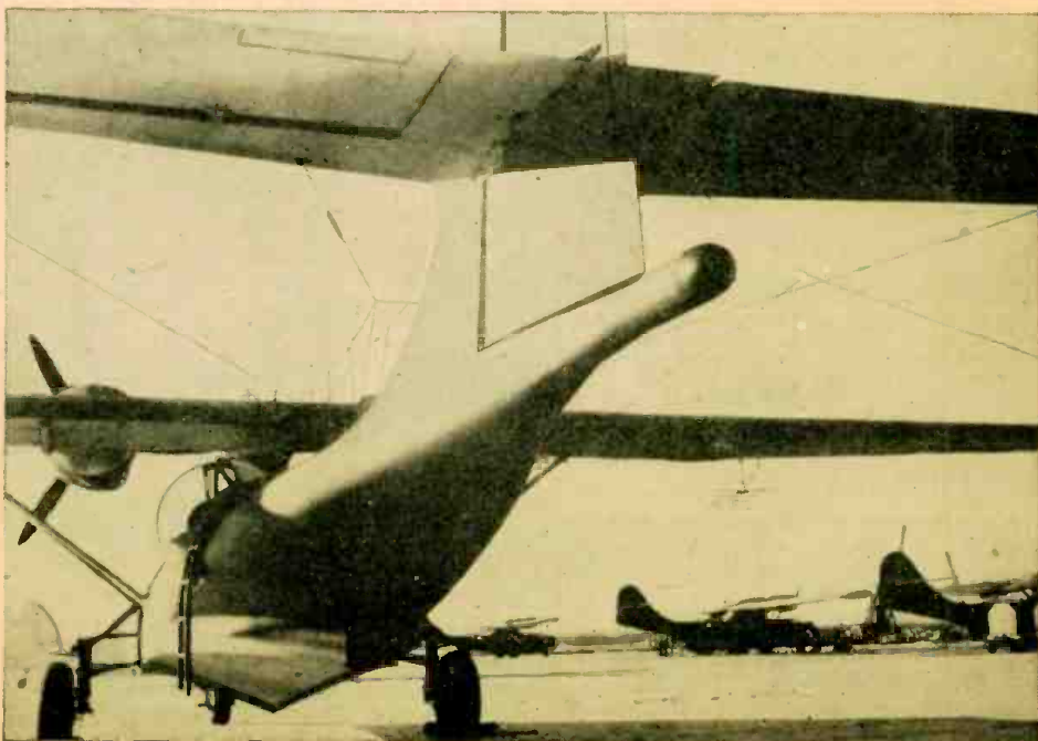
The "doodlebug" is carried in the rounded cylindrical projection at the tail of the plane.
