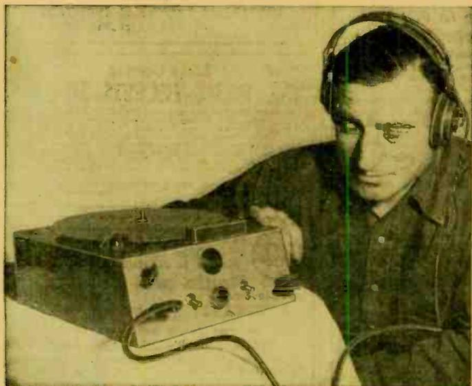
This interesting code teacher uses a disc of the old Omnigraph type which sets up any one of four tones, works a mechanical key to give the student the "feel" of the code, projects dots and dashes on a transparent dial and flashes a blinker at the same time. By thus co-ordinating all the senses, learning time is cut down, reports Harold Herman of Chicago, its constructor.
