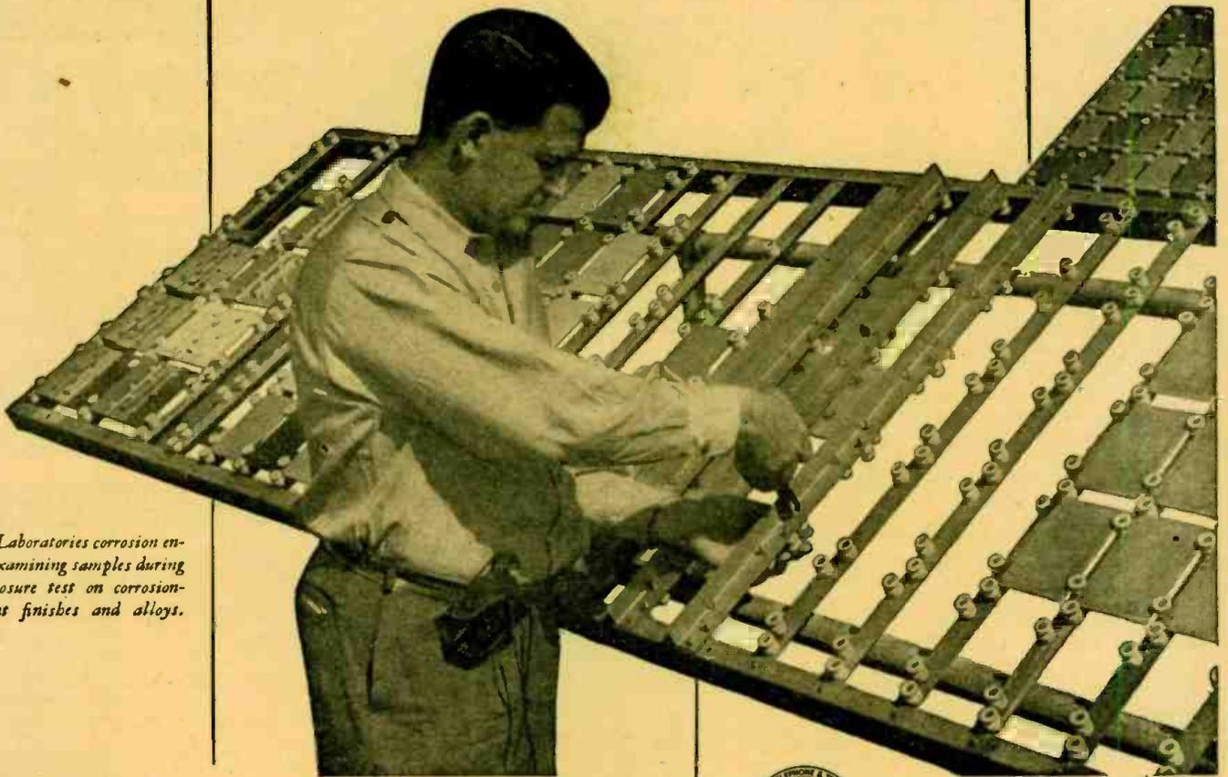
*A Bell Laboratories corrosion engineer examining samples during an exposure test on corrosion-resistant finishes and alloys.*
