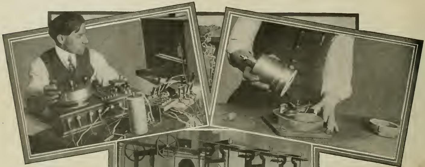
The Above Illustrates One of Uncle Sam's Coal Testing Experts Operating an Electric Resistance Bridge Connected With the Bomb Calorimeter.
