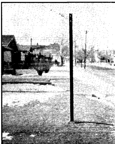
ANCHOR POSTS FOR GUYS AS DESCRIBED IN THE TEXT
